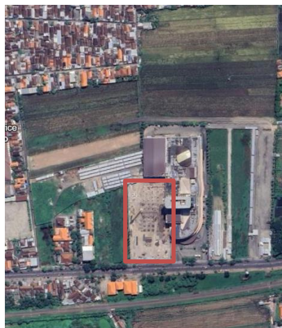
Figure 1. Site plan for the construction of Sunrise Mall 2 in Mojokerto City ( https://earth.google.com , 2025)
